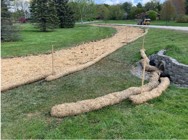
29 Gundalow - 1 (Drainage Area)
