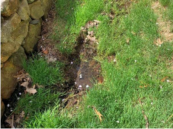
4 Brickyard Circle – 3 (Drainage Course)
